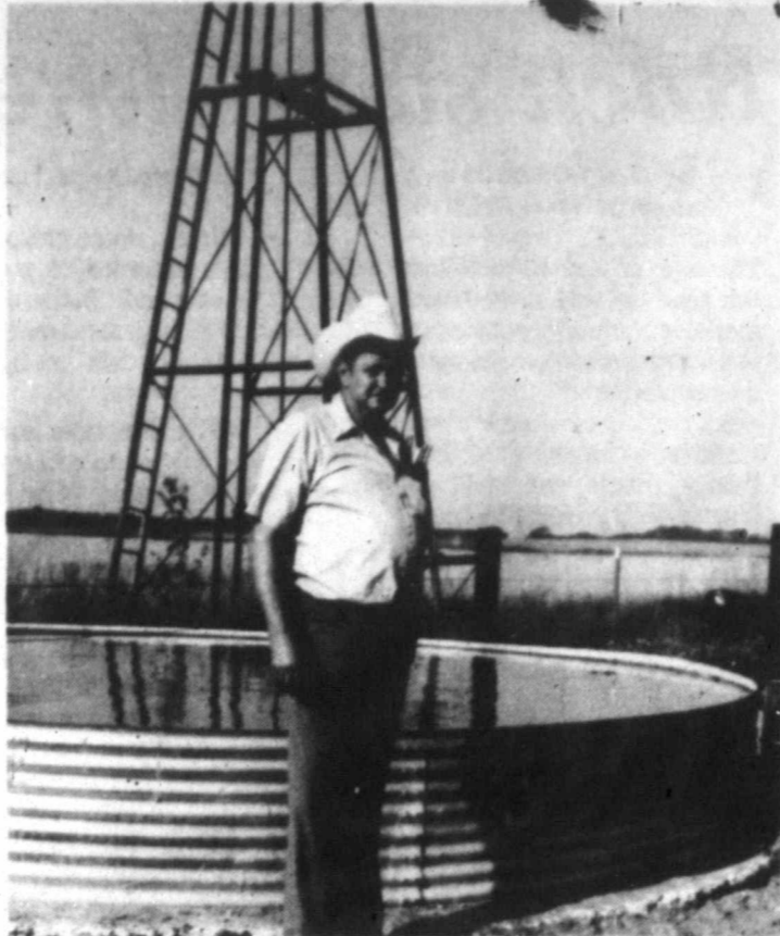
Water well added
