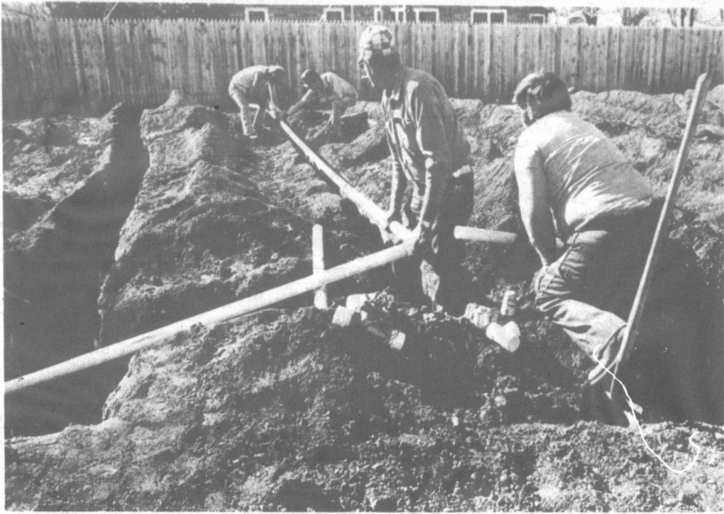
Installing sprinklers
