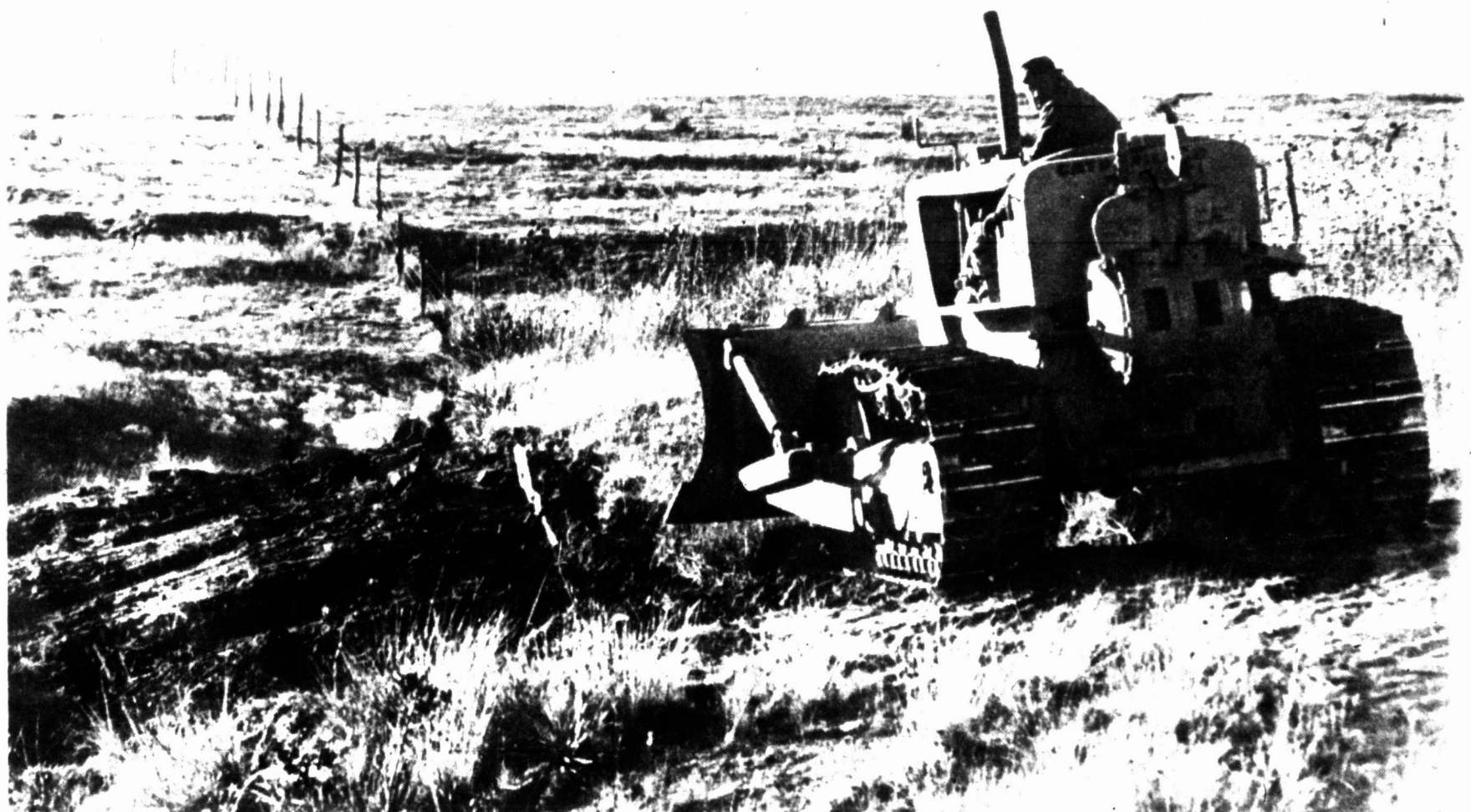
Sewage Plant Beginnings
