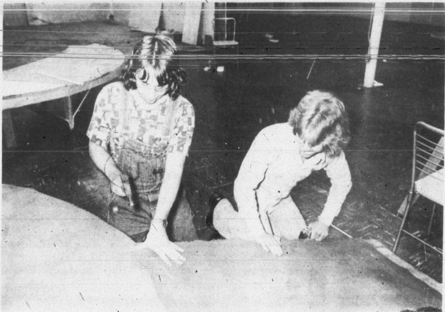
Stage Center Ronnie Holmes and Ocie Powell try their hands at carpentering as they work to transform the Shoeland Building into a community theater for Pampa. The newly formed group plans to put on the musical, "The
