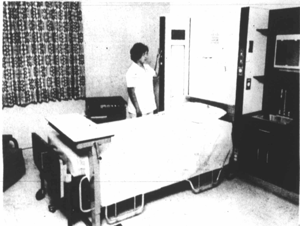
HILL-ROOM Enviro Care Units in 99 new patient rooms in St. Anthony's Hospital, Amarillo, are complete modules containing closet, basin, cabinets, and console-control of lighting, color television, telephone, and other functions.
