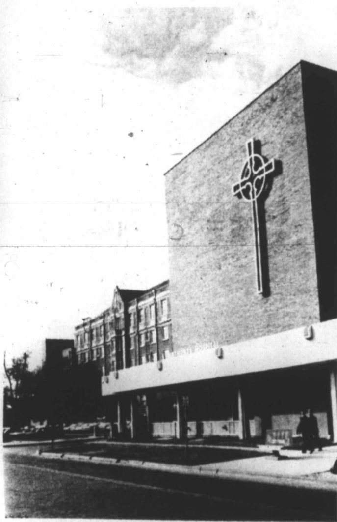
THE ORIGINAL WING of St. Anthony's Hospital, known as Annex B, is shown on the left. The red tile roof has been an Amarillo landmark for half a century.
