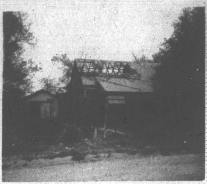
PUBLIC EYEBROW — If you remember seeing this tumbledown house at 313 W. Tuke, it's not there any more. It is one of many unsightly abandoned structures being torn down and hauled away in the city's continuing campaign to remove landscape eyesores. Only recently the same thing has happened to old buildings at 421 Harlem, 408 Harlem, 528 Oklahoma, 546 Elm and 626 Elm.
