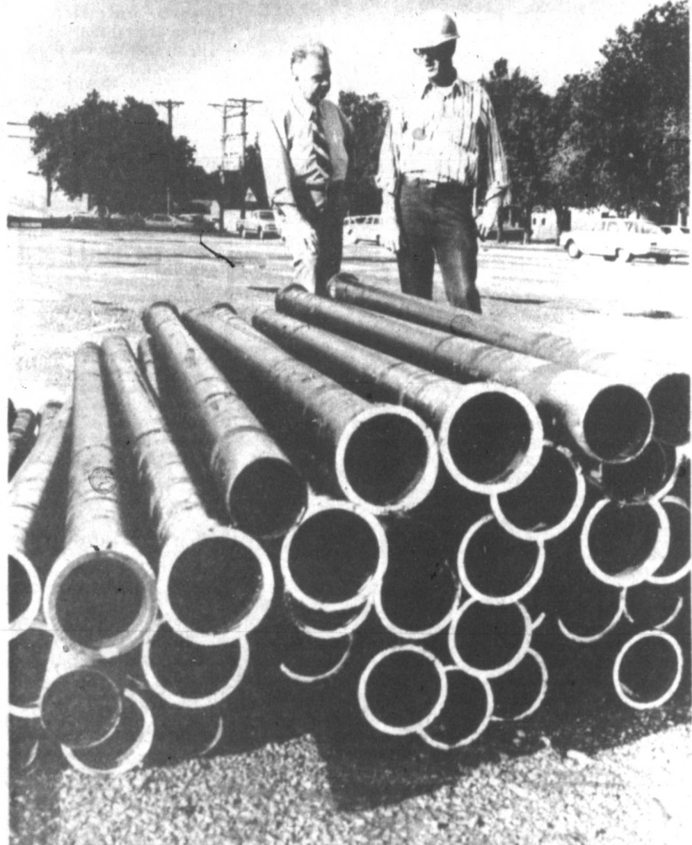
GETTING IT ORGANIZED—Cameron Marsh, principal of Pampa High School, left, and Wallace Birkes, superintendent of Wiley Hicks Construction Co., look over a set of pipes to be used during the construction of the new vocational-technical building at the school. Officials and contractors developed the layout this week. Excavation for the site is due to begin Monday for the new addition to the campus. (Staff Photo by John Ebling)
