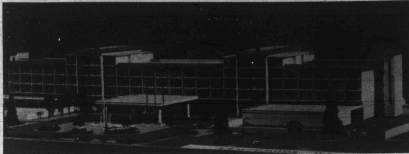
BROADMOOR WEST — From a west side entry drive, portrayed in this Broadmoor West replica, guests may park in private areas, register in the lobby and take any of four elevators to their air-conditioned rooms.
