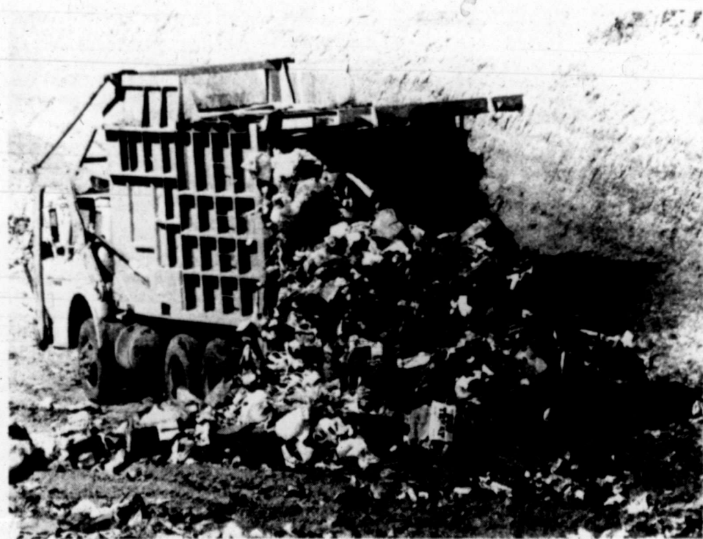
TRUCKS DUMP THE TRASH IN A CUT AT THE LANDFILL
