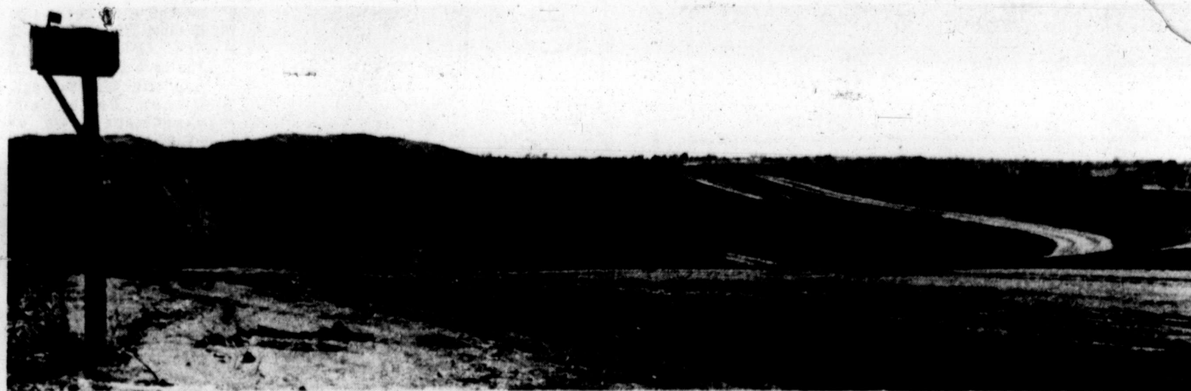
THE CUT IN THE RIGHT PORTION OF THE ABOVE PHOTOGRAPH WILL BE BUILT UP TO LOOK MUCH LIKE THE FINISHED FILL AT LEFT
