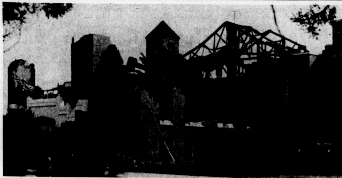
WALLS COME TUMBLING DOWN — Moving towards construction of the new auditorium and offices for First Baptist Church, Wilson Salvage Co. of Lubbock has been tearing down the old structure destroyed by fire last December. The
