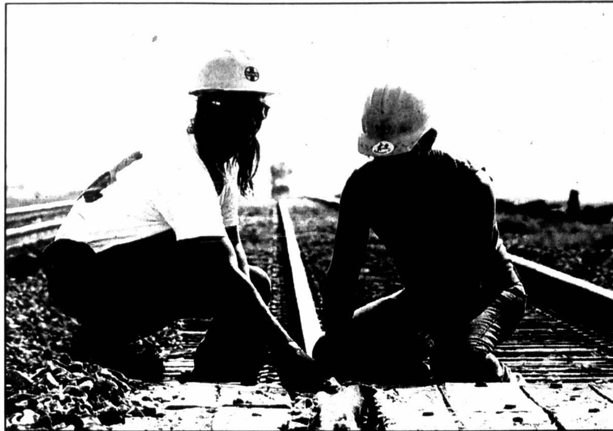
Tie gangs, surface gangs and road crossing gangs were out between thunderstorms this week performing planned maintenance on Santa Fe Railway lines from East Pampa to Pantex in Carson County. The maintenance project that has been scheduled for five years is not quite half way through, according to railroad officials. More than 100 men are involved in the project including R.W. Hill, left, and Fred Manly, both from Arkansas City, Kan., who were working on a crossing near White Deer Monday afternoon.
