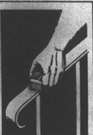
SANDPAPER RUSTED AREAS.
