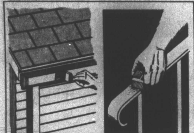
APPLY ZINC-RICH PRIMER TO GUTTERS.
