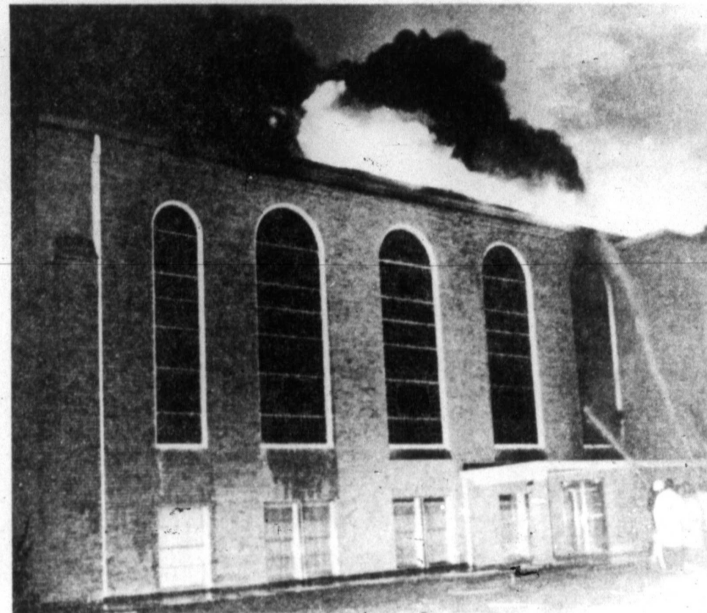
A DESTRUCTIVE FIRE destroyed parts of First Baptist Church in December
