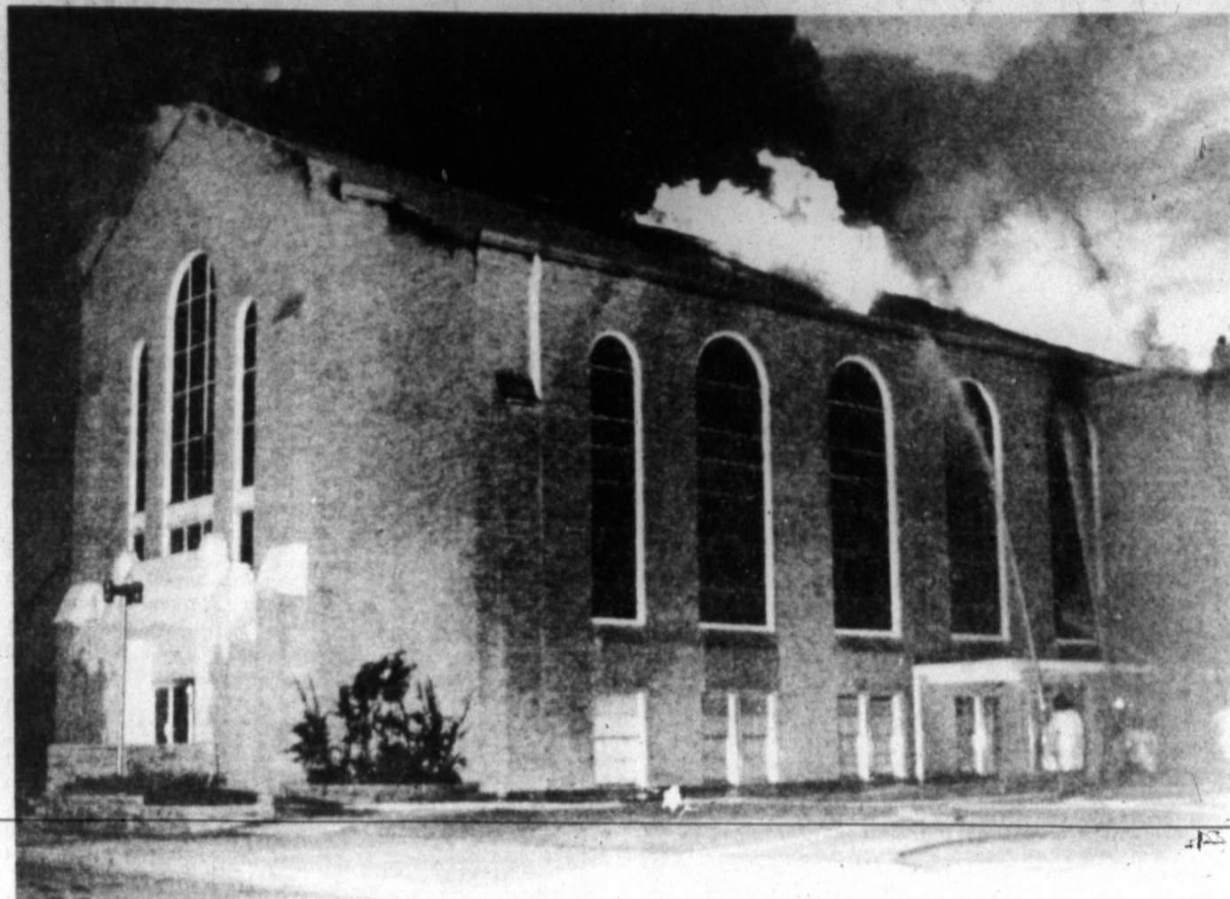
FIREMEN battle the blaze as it breaks through the roof
