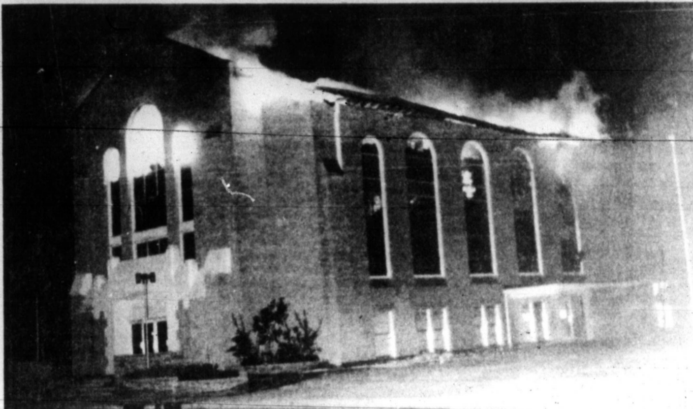
CHURCH ABLAZE — The First Baptist Church, 203 N. West, suffered extensive damage to the sanctuary and parts of the education building as a fire roared through the structure Sunday afternoon and into the night. Rev. Mr. Claude
