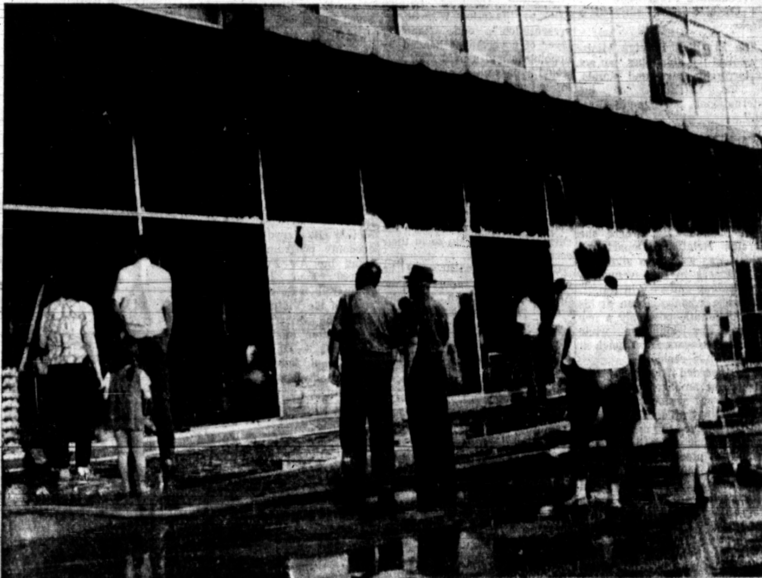
AFTERMATH OF the half-million dollar fire that ravaged Furr's Food Store in today's early morning hours, attracted sidewalk spectators throughout the morning. Some had come with grocery lists in hand, not knowing of the fire; others to speculate upon the fire-blackened merchandise and the collapsed roof at the back of the store just above the frozen-food and meat departments. (Staff Photo)
