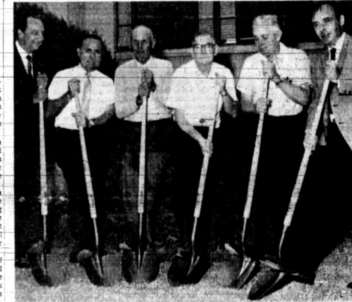
HIGHLAND GENERAL Hospital Board of Directors broke ground Thursday for the remodeling and construction program which is scheduled to begin Aug. 27. From left are E. L. "Smiley" Henderson, Wes Langham, hospital administrator, O. R. Blankenship, Joe Miller, Gordon Lyons, chairman of the board and Gene Imel, secretary.
