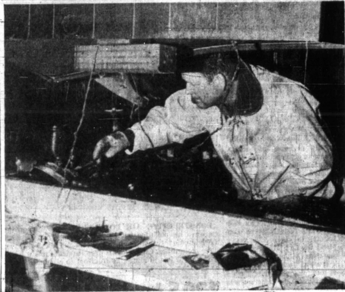
INSPECTS FIRE DAMAGE — Pampa Fire Department Captain Al Ferguson inspects heavy damage sustained by the kitchen of a trailer home owned by Wayne Caudell, Pampa Trailer Park, after a fire broke out late Thursday afternoon. The remainder of the trailer suffered smoke damage. Cause of the fire has not been determined. (Photo By Bob Kelly)
