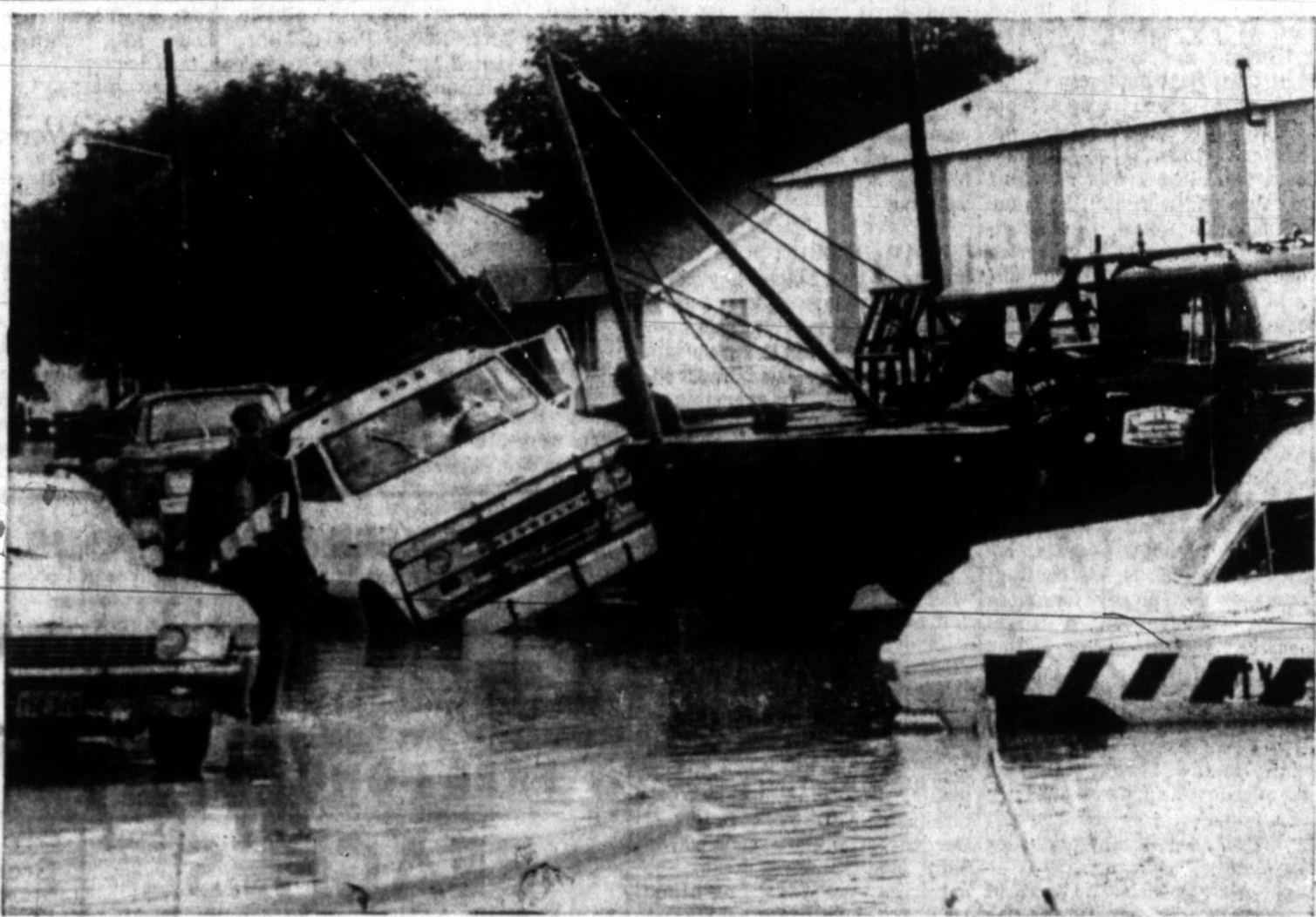
THAT BARRICADE WAS A LITTLE LATE—Cars and trucks had a hard time getting around the intersection at Barnes and Frederic Tuesday morning as hard rains hit Pampa. The biggest trouble was caused as rain washed out the base from a newly completed sewer line which cuts across Highway 60 at the intersection. Several cars and trucks, including a police car sent to the scene to control the traffic, fell victims to the trench. City crews were working hard to replace the base over the line and get the intersection open by noon.
