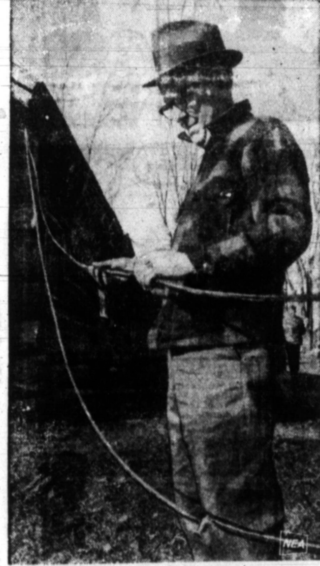
NEW APPLICATION for an established principle may quadruple maple syrup production, according to Vern Folt, seen here watching sap flowing uphill through plastic tubing. Folt, a dairy equipment expert from Burton, Ohio, wondered why a vacuum pipeline system used in milking cows couldn't be applied to the gathering of maple sap. This year, he ran tubing from a compressor in the sugar shack to the trees and back. He reported great success and farm agents estimate the system could move more than 300 per cent more sap than previous methods.
