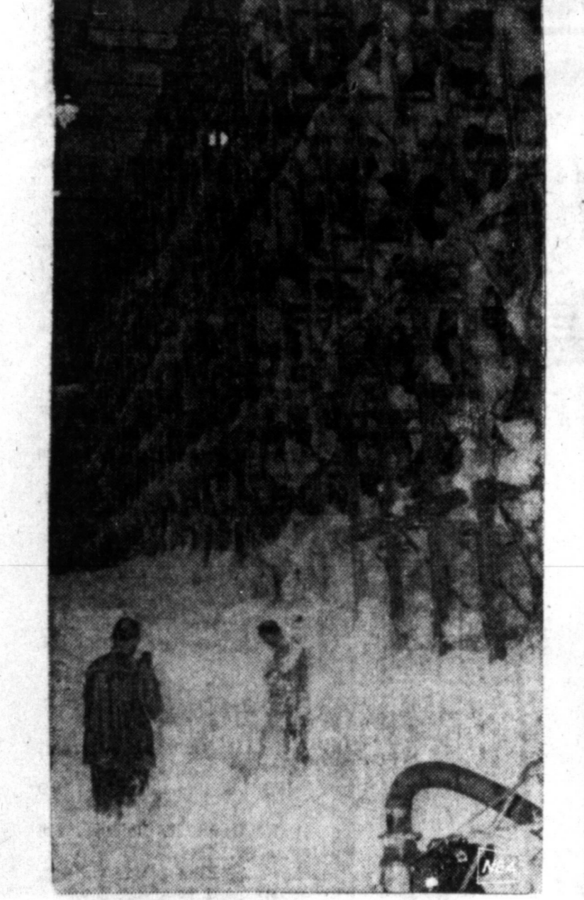
INDOOR BLIZZARD? From the looks of things, someone forgot to shut the doors of this warehouse during a snowstorm. Actually, the white stuff is detergent foam generated by a new fire-protection system. In a recent test, the 60-foot-high, 8,000-square-foot building was filled from top to bottom in seven minutes. Because foam smothers fire quickly and its low water content minimizes stock damage, the system was installed at Ford's Fostoria, Ohio, plant.
