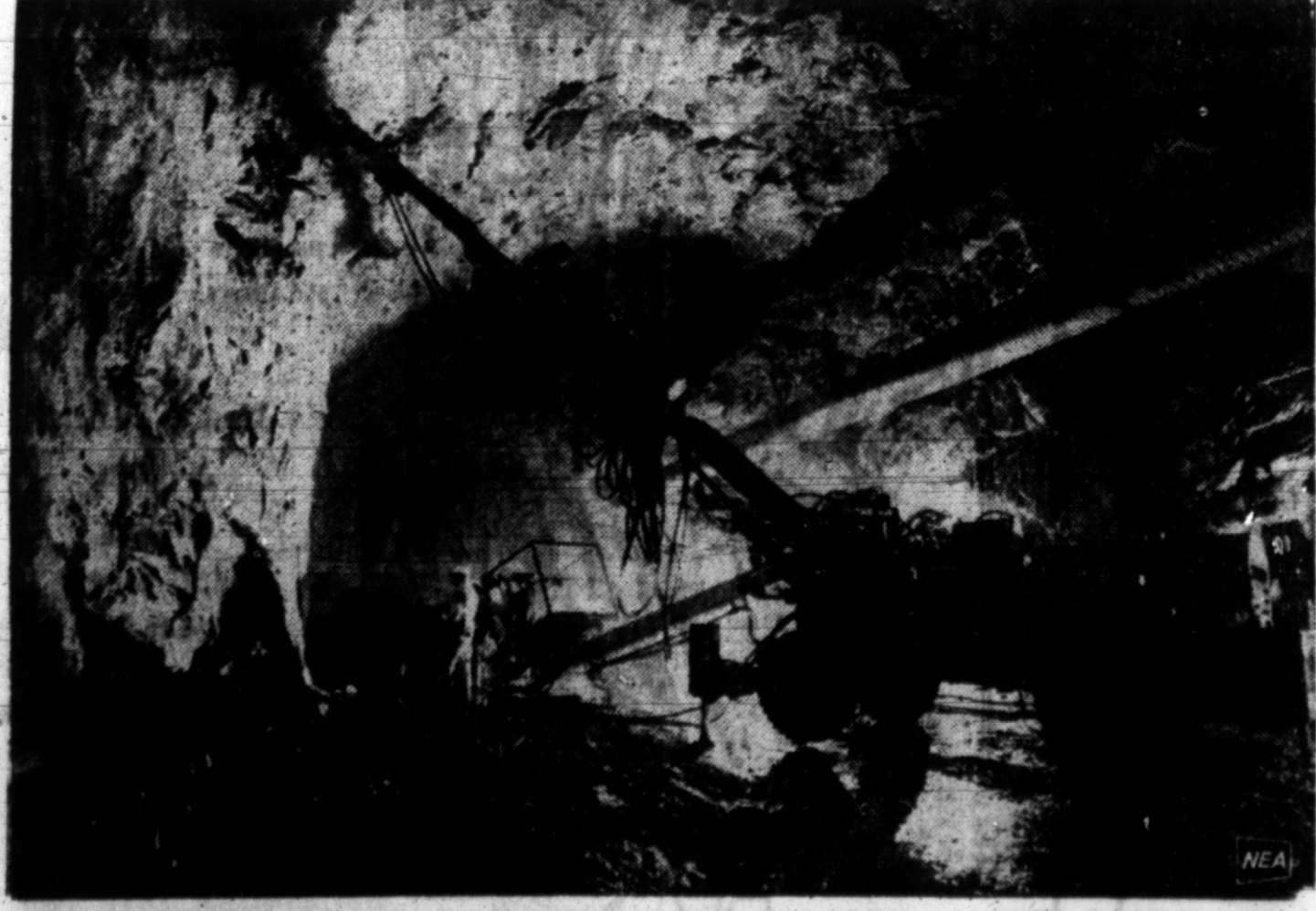
AFTER BLASTING through a mile of solid granite, workmen are carving this huge cavern deep in a hillside in New England. It and two similar chambers will be part of the Churchill Falls hydroelectric project scheduled for completion in 1976. Operations have been underway since 1966 on the massive enterprise.
