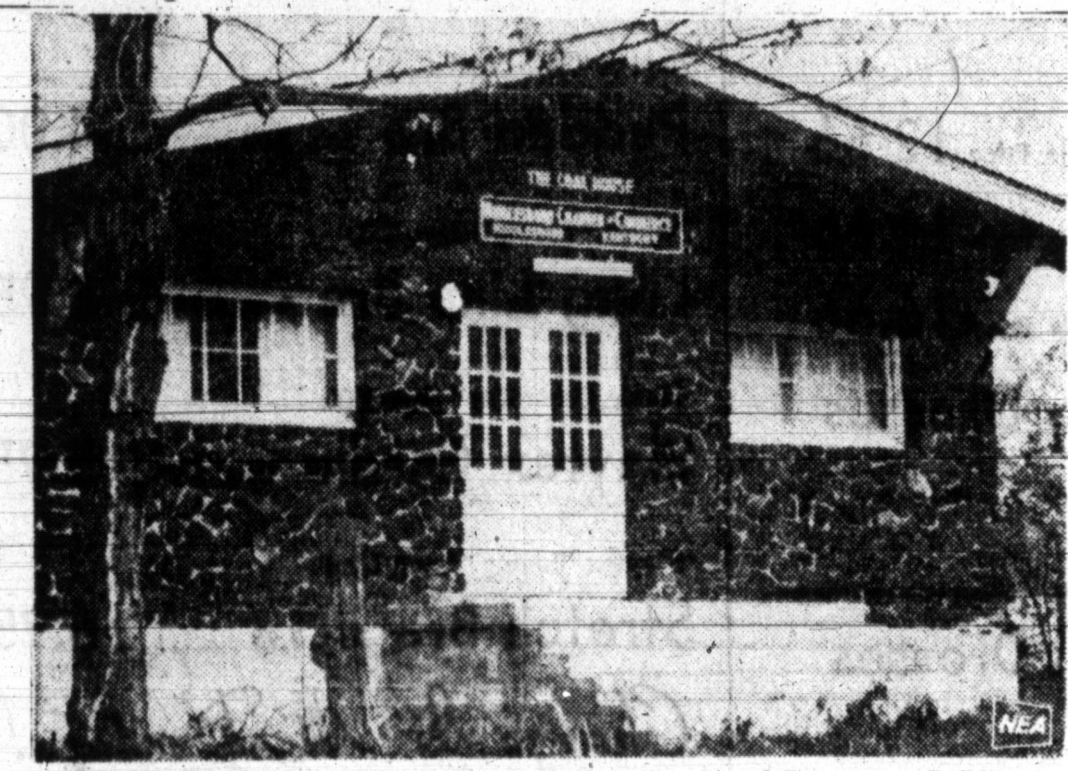
COAL HOUSE is home to the Middleboro, Ky., Chamber of Commerce. Building is one of the few in the United States to be made of coal. Officials used the unusual building material to promote the image of coal in the area.
