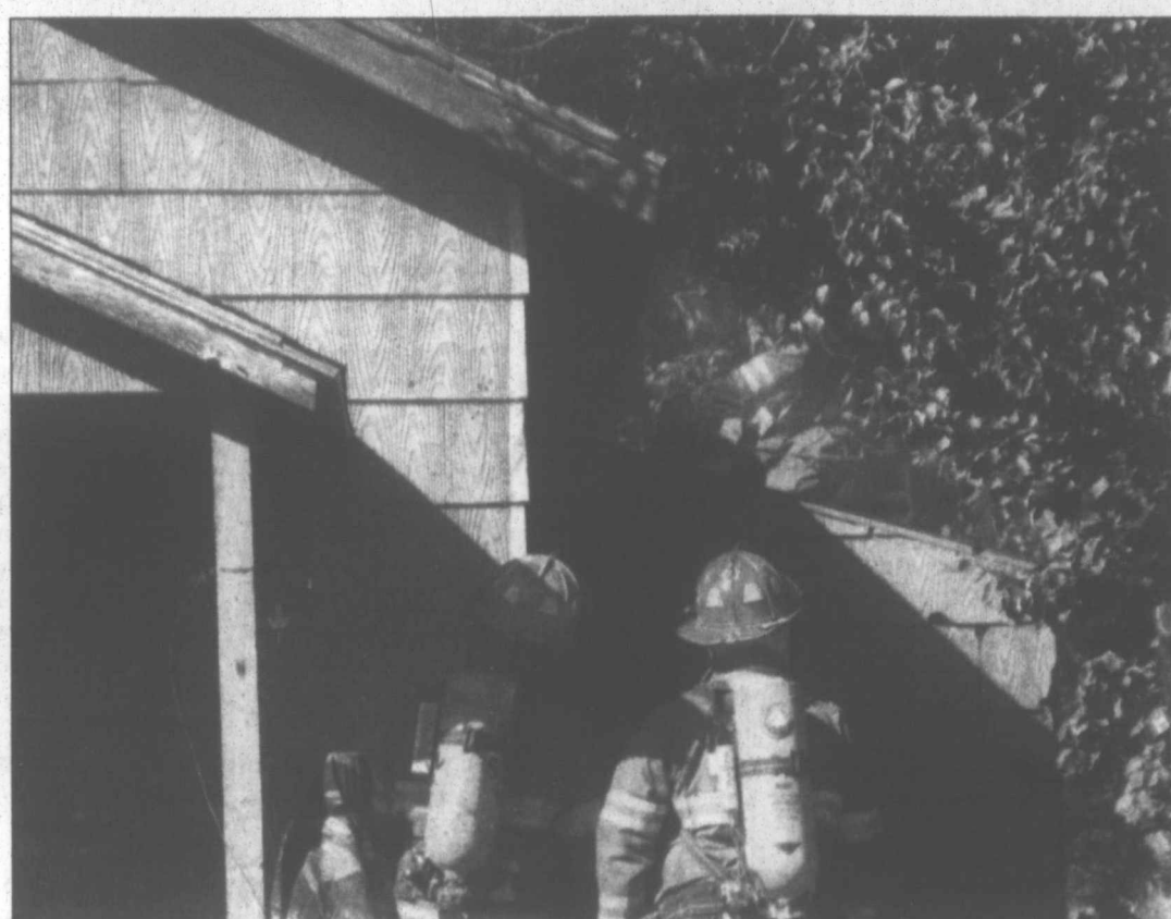
staff photo by Julie Ann Thompson A space heater was the cause of this house fire yesterday in Pampa.
