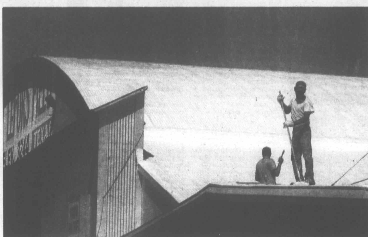
Pete Rodriguez with Crawford Roofing puts a coat of polyurethane atop the Perry Lefors terminal. Bob Crawford, owner of the roofing company, said the new coating, when it's finished, should provide insulation, water proofing and wind resistance for the terminal and main hangar.
