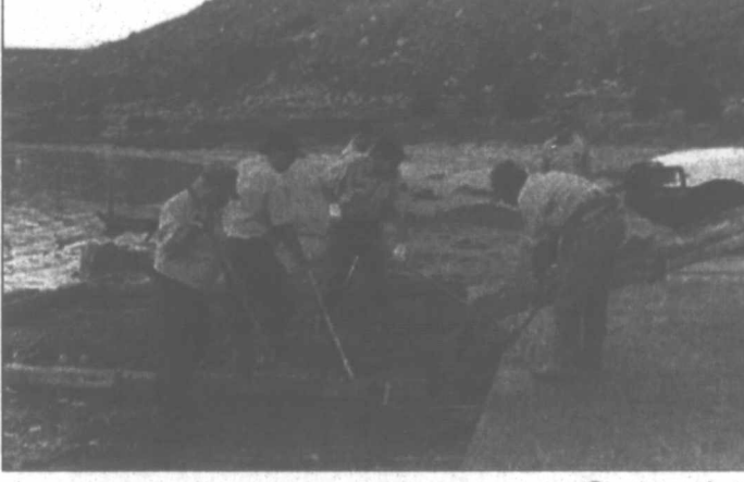
Concrete is poured at Fritch Fortress last week.
