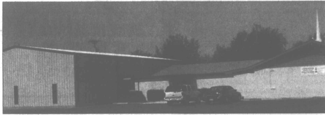
A new larger sanctuary, left, is almost complete for Lighthouse Covenant.
