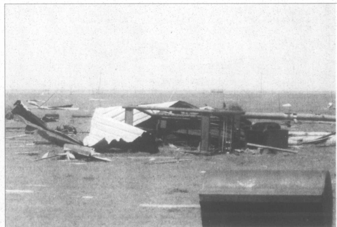
Metal sheeting is wrapped around metal pipes.
