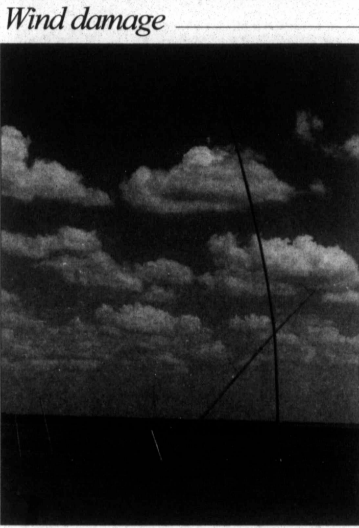
Wind damage Pampa News photo by MARILYN POWERS An antenna located on Highway 152, one mile east of the Highway 152-Highway 60 split, was reduced recently to a snarl of antenna segments and guy wires, possibly due to strong winds. No high winds are forecast this week, and any current threat to property will likely be from flash flooding due to continued heavy rains.
