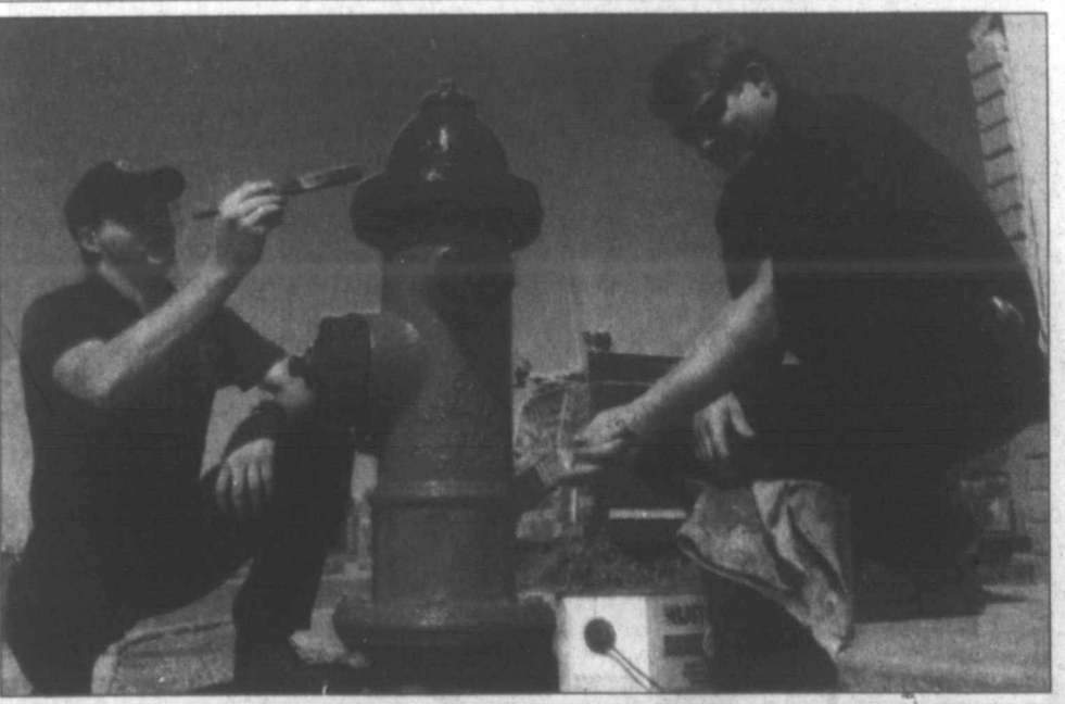
Pampa News photo by DAVID BOWSER Kasey Presson, left, and Bob Griffin do some routine maintenance on a fire hydrant at Gray and Brown Monday. They will participate in an international stand down Wednesday to concentrate on safety issues.
