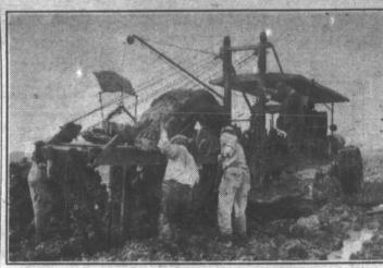
Huge ditching machines go deep and wide to make more room for oil and gas pipe lines throughout the Panhandle oil and gas field. Above is a machine in action, plowing through mud preparatory to the laying of pipe through which gas or oil flows hundreds of miles. Pipe lines from 6 inches to two feet in diameter lead out of the Panhandle
