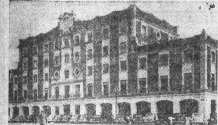
When the Mexican government confiscated oil properties in Mexico it expropriated everything it could lay its hand on. Above is the British oil building, just completed at a cost of $600,000, which the government promptly took over as headquarters from which to administer the confiscated oil wells, derricks and pipe lines.
