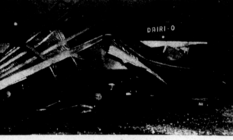
McLEAN STORM DAMAGE Residents of McLean and nearby Heald, slashed late Monday by heavy rains and a tornado respectively, were still counting their property damage today. Pictured here is the toppled and bent tin canopy of the Highway 66 Dairy-O, owned by Bob Taylor, in McLean. At left in background is an overturned trailer house. McLean received four inches of rain during the Monday storm. (Photo By J. M. Payne, McLean)
