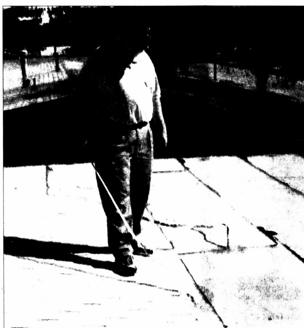
(Pampa News photo by Marilyn Powers) Ronnie Parsley of Double D Roofing inspects hail damage left by a severe thunderstorm which hit Pampa on the evening of June 21. This roof is in the 2300 block of Rosewood.
