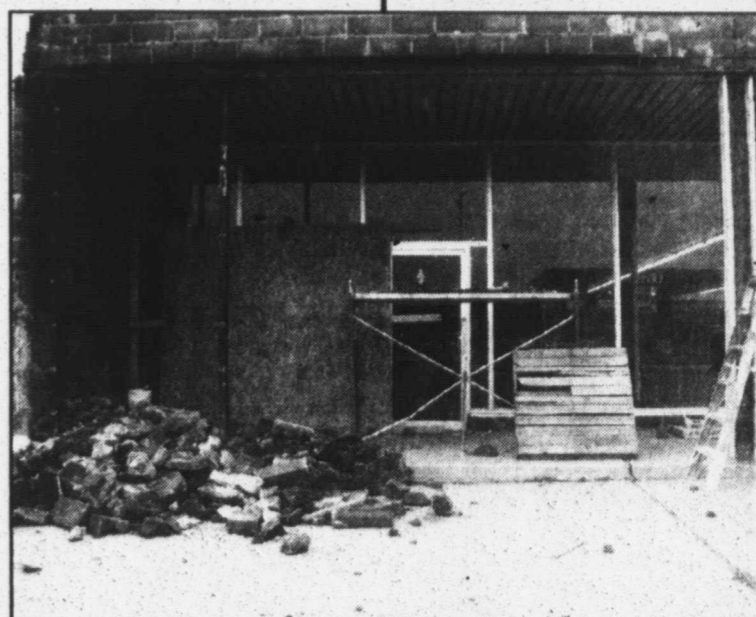
Renovation continues on the future home for Texas Furniture.
