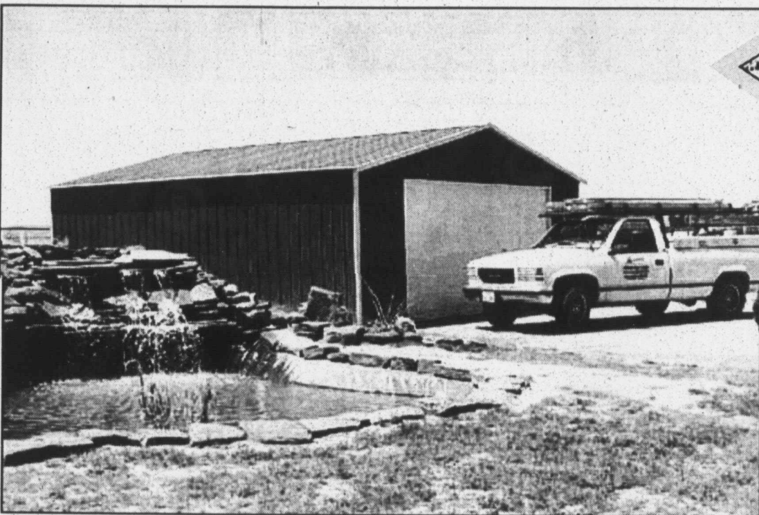
▲ Rasco Construction's custom-built buildings are of varying sizes and designs. The staff builds any size custom building to the specifications of the customer.
