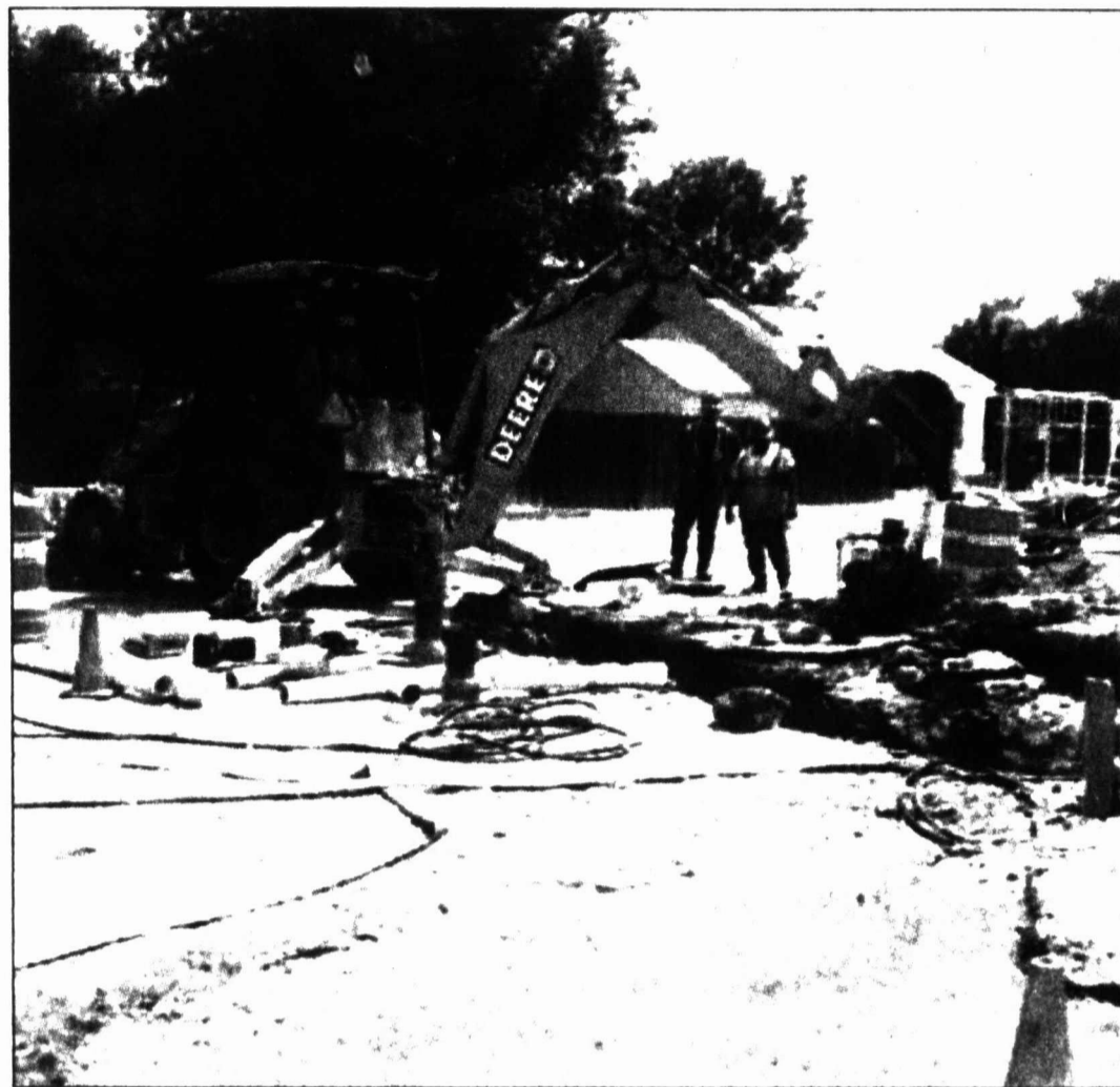
(Pampa News photo by Dee Dee Laramore) City of Pampa workers, from left, Ron Parnell, Andy Werner and Michael Campos, repair a four-inch water main that burst Tuesday between Lefors and Magnolia streets. When city employees arrived at the break, a stream of water was shooting high into the air and gallons of water rushed down Magnolia and continued down Browning Street. Parnell said this is the fifth water main that's broken in the city in the past three days. Residents on the north end of the two residential streets were without water until workers could repair the line.
