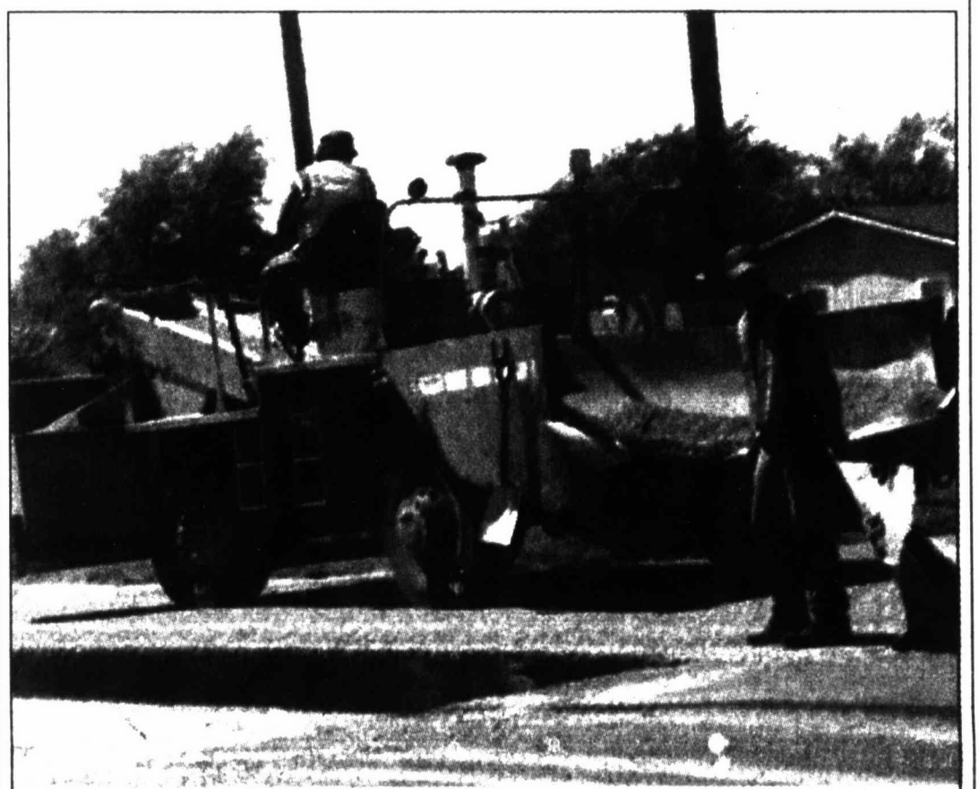
(Pampa News photo by Skyla Bryant) A crew from Lewis Construction Company of Dumas uses a chip spreader to lay asphalt and gravel at Wilks and Barrett streets Friday afternoon. Terry Brown, crew chief with the City of Pampa, said the work is part of the city's annual seal coating program now under way in several areas of town.
