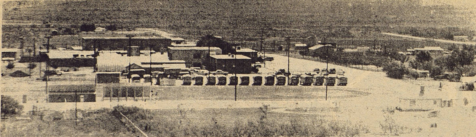
GAIL CAMPUS — Seen from the caprock, the Borden County High School and all the support buildings appears to be almost a community in itself. The school is located near Gail.
