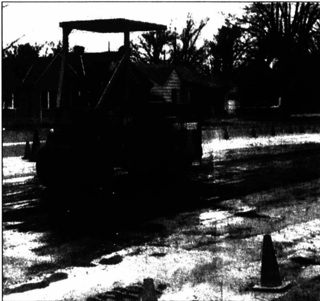
(Pampa News photo by Dee Dee Laramore) City of Pampa employee, Morris Long, uses a steam roller to smooth out a patch on Somerville Street Wednesday afternoon.
