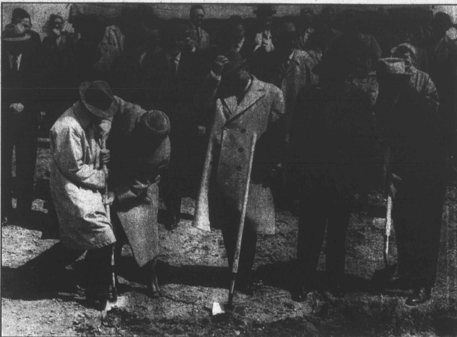
(Pampa News archive photo) Groundbreaking for the Pampa Community Hotel took place this morning (April 21, 1959) under a chilly April sun, but the exuberance of the five official ground breakers did much to warm the occasion. Left to right, the official turners of the soil are C.P. Buckler, Inez Carter, George Cree Jr., Mayor Ed Myatt and Chamber of Commerce President Warren Hasse. The team of Buckler-Carter on Shovel No. 1 seemed to have the edge on all comers. When the ground breaking was completed for spectators and cameramen - who always need "just one more shot" - a ditch of surprising size had been dug.
