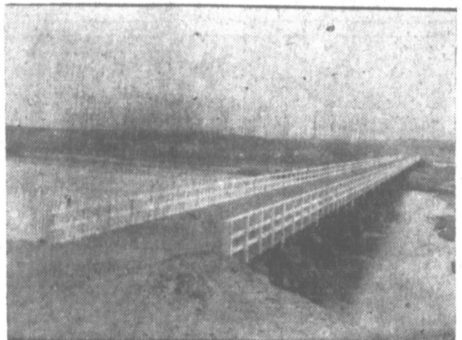
Most prolific of recently discovered pools in the Panhandle oil field is the "hot spot" of eastern Gray county and west central Wheeler county. Pictured above is the bridge which Gray county built over the treacherous McClelland creek for use by the oil men. (NEWS Staff Photo and Engraving.)
