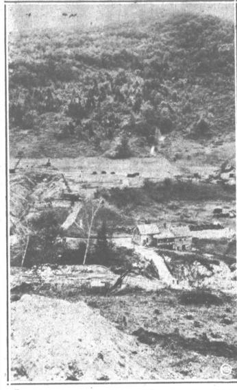
Daming of the Little River in Vermont's Green Mountains, which has just been started, is the largest flood control project in New England. Steamshovels are shown at work preparing excavations for the dam The project, to cost \$5.000 000, is designed to prevent the
