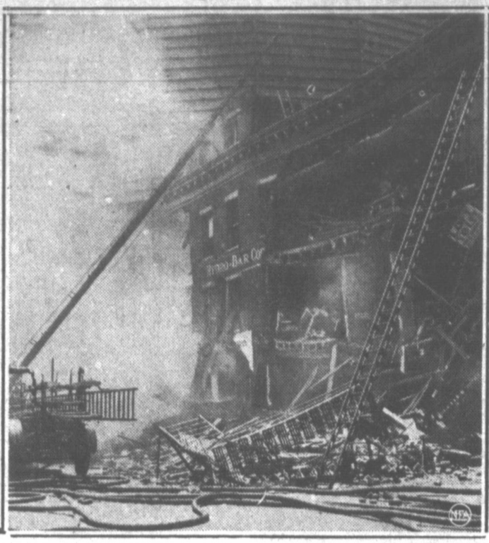
An explosion in an automobile service station caused one of the most serious recent tragedies in New York, burying a half dozen occupants of nearby buildings in the debris of their wrecked homes
