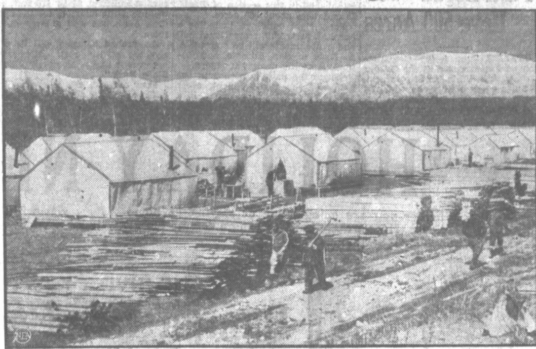
Housing the 500 midwest families colonizing the Matanuska valley in Alaska, this tent city teems with activity as the pioneers, aided by details of transient workers, build their homes, clear the timber, and prepare the land for their first crop next year. Soaring back of the picturesque town of canvas are the snowcaps of the Chugach mountain range, a vivid contrast to the fertile valley where the sun now shines until nearly midnight.
