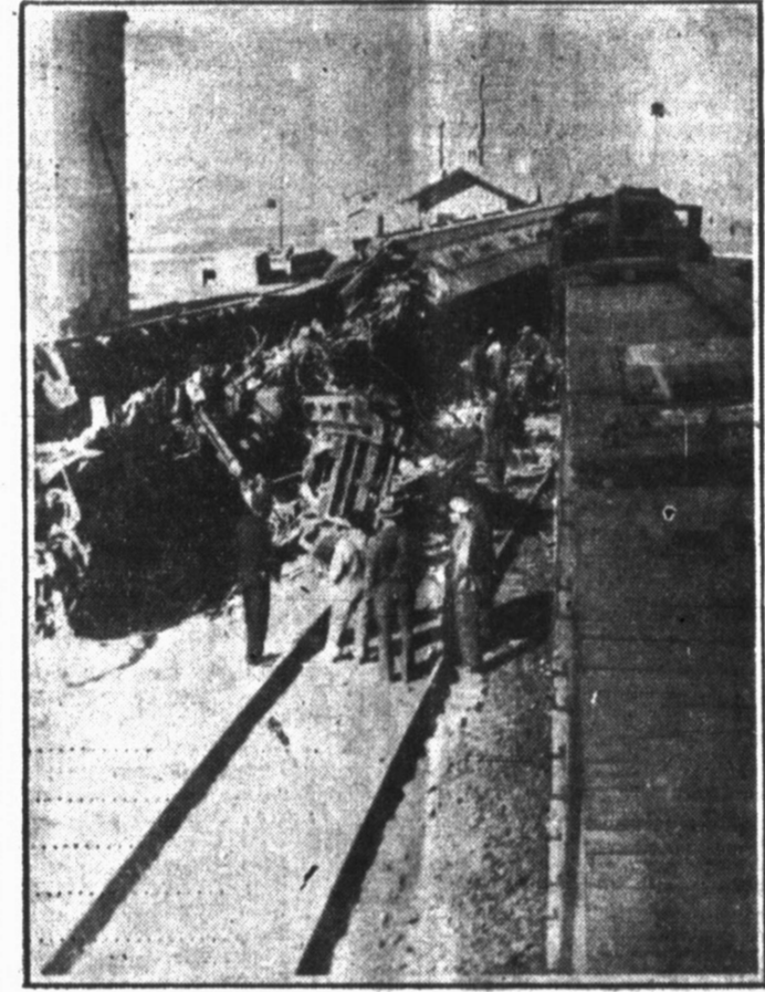
Before a special passenger train bearing CCC workers from Oregon to Fort Sheridan, Ill., could clear a siding Tuesday morning at Shields, Kans., a fast Missouri Pacific freight, westbound, ploughed into the two rear tourist Pullmans of the special. Thirty CCC workers were injured. The above photograph shows the two wrecked Pullmans and, at the right, the freight train. (NEA Photo.)
