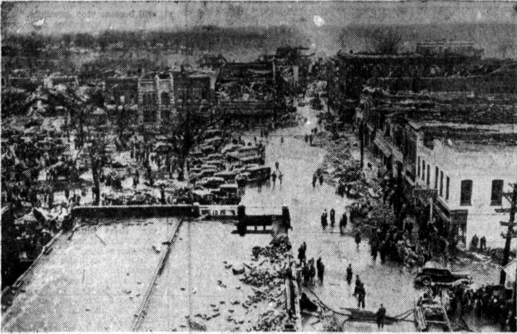
Gainesville, Ga., April 3, 1936—Battered by the full fury of a tornado that claimed 200 lives, the Public Square of Gainesville, above, was filled with debris after storm and fire had taken their toll. Within the city limits 922 structures were damaged; loss was estimated at more than $10,000,000. Only the statue of a Confederate veteran, standing in the middle of the square park, escaped unscathed. Ambulances, fire trucks and rescuers' automobiles crowded the chaotic scene as throngs of survivors picked their way through the wreckage.
