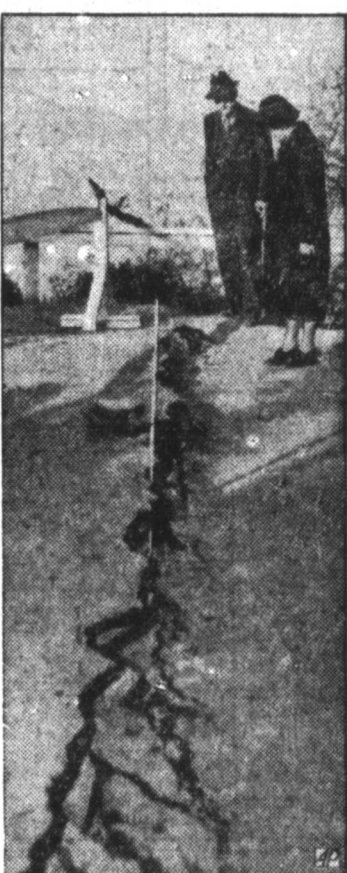
THE BAD EARTH of a 400-foot bluff, slowly settling at Elysian Park, Los Angeles, caused this crack and fears of a landslide.
