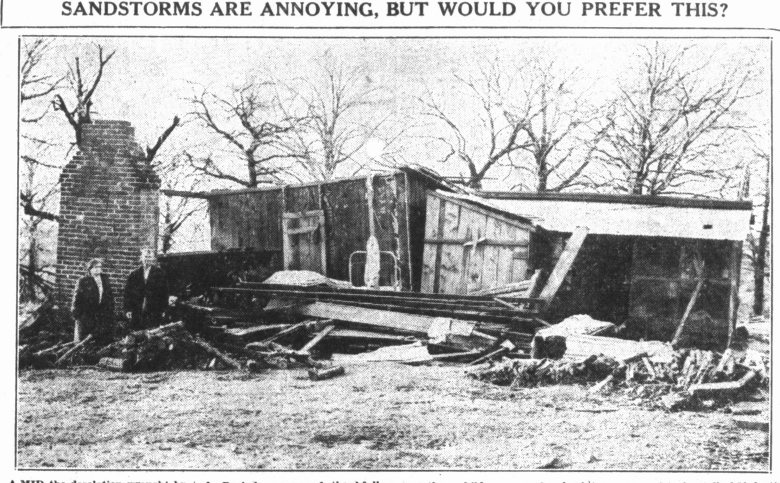
A MID the desolation wrought by cyclones that cut swaths through four southern states, Mr. and Mrs. A. Buckalew surveyed thankfully the wreckage of their home near Mount Sylvan, Texas. The couple and three children escaped unhurt when the frame structure crumbled in the cyclonic fury, that killed two persons and took a toll of 81 deaths in Texas, Arkansas, Mississippi and Louisiana.
