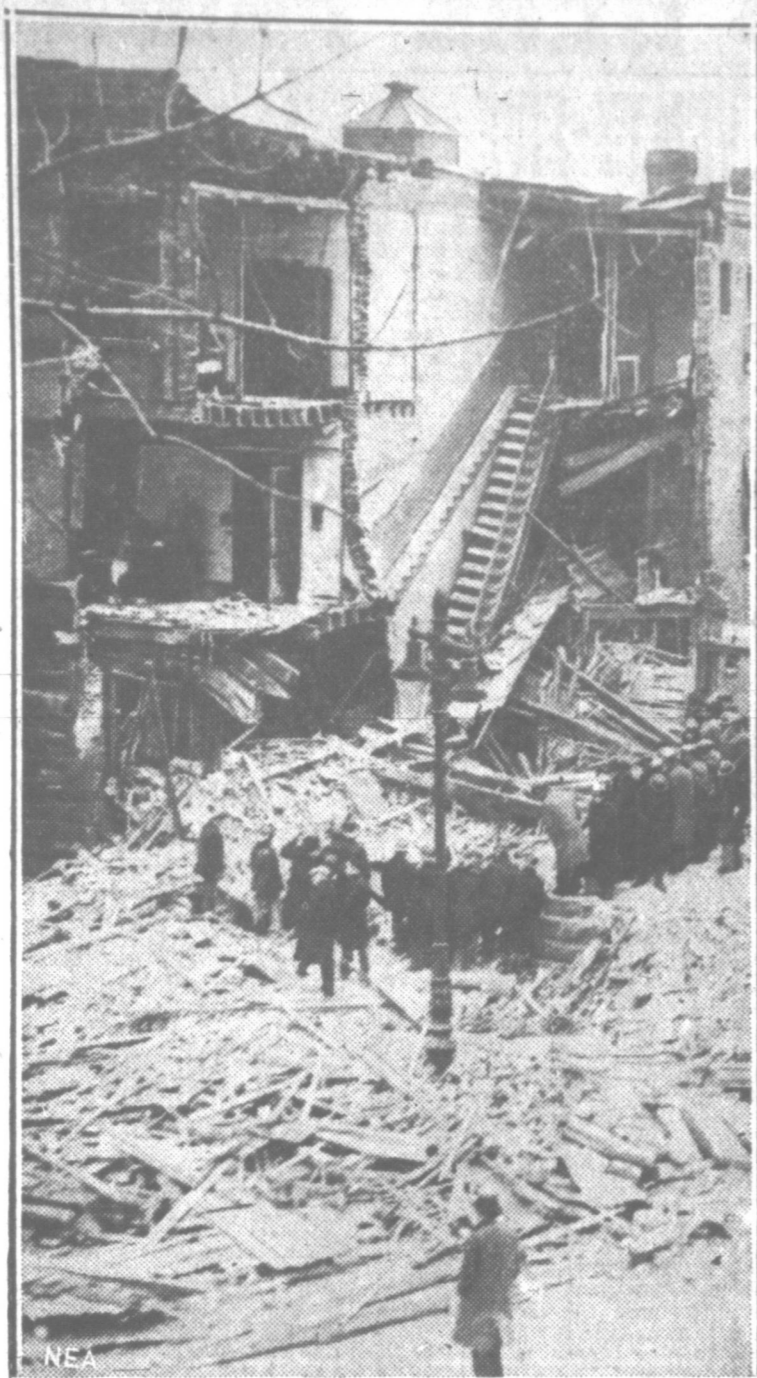
CONVINCED that only a bomb could have brought about the destruction pictured here, Philadelphia police sought clues to an "inspector" believed to have planted an explosive in the home of John M. di Silvestro, banker and national head of the Sons of Italy. Di Silvestro's wife was killed and sixteen persons were injured in the wreckage of the three-story house.
